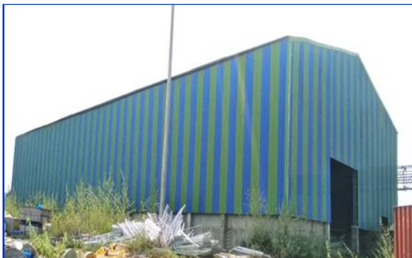
Closed sheds for Raw Materials
