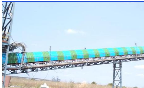
Closed Conveyor Belts for Limestone
