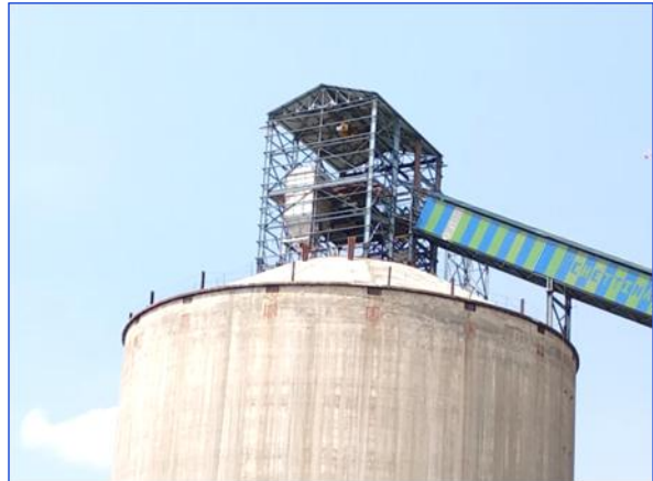
Bag Filter at Clinker Silo top
